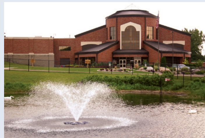
Eden Prairie Water Treatment Plant
